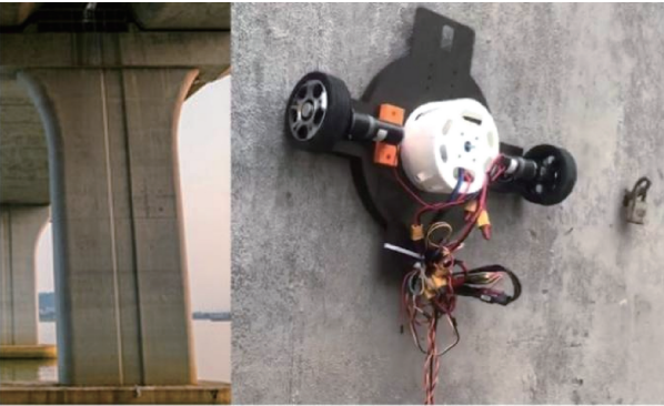
(a) 待检桥墩 (b) 机器人本体壁面吸附 (a) Inspecting bridge piers (b) Robot adhered to the wall surface
