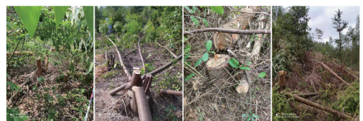
(b) 配电网树障清理工程场景 (b) Detection scene of tree barrier clearance workload
